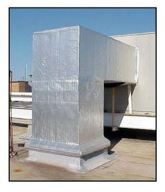
**Alumaguard® Lite** flexible weather-proofing cladding from **Polyguard Products** is one of the family of **Alumaguard** cladding products that offers superior cold weather performance, ease of handling and application and true zero perm performance
