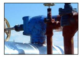
**RG-2400 LT** is a surface conversion compound utilizing mineralization technology, or the "science of Minetics"; this compound replaces the corrosion process with a mineral formation on and into the metal creating a mineral barrier 50-200 angstroms deep into the metal surface.
