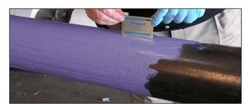
**RG-2400 NP** is an anti-corrosion gel utilizing Polyguard's mineralization technology, (the "science of Minetics"); this gel replaces the corrosion process with a mineral formation on and into the metal surface creating a mineral barrier 50-200 angstroms thick. A pH in the alkaline range passivates water vapor, and the hydrophobic nature of the gel repels water.
